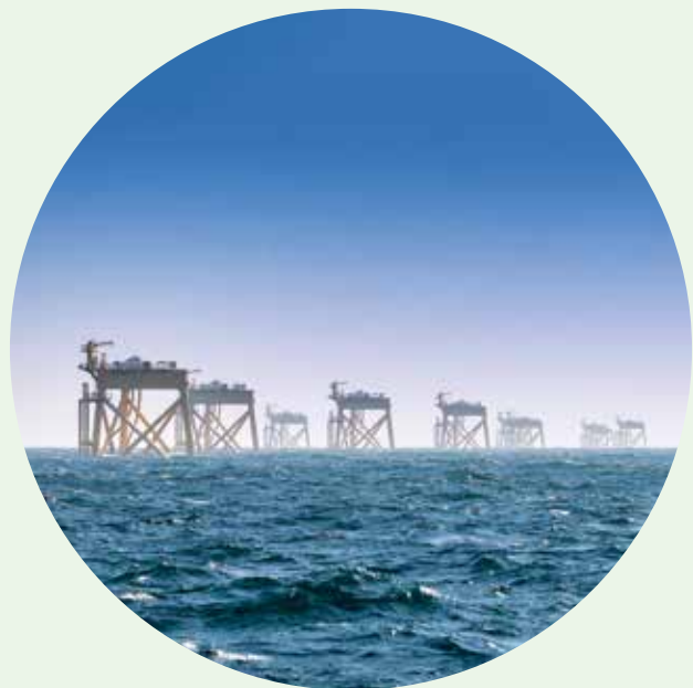
©ScottishPower Renewables Jacket foundations installed
