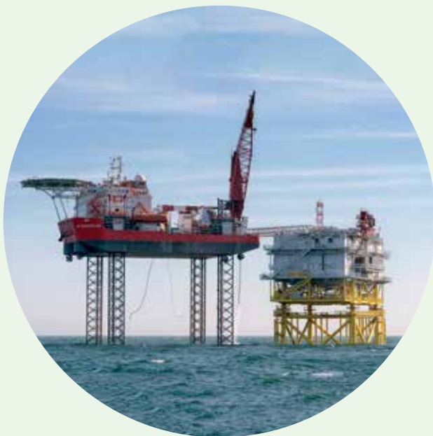
©ScottishPower Renewables Offshore substation and GMS Endurance jack-up accommodation vessel.
