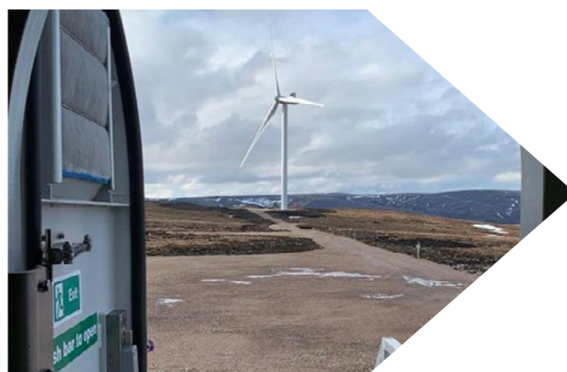
Nanclach onshore wind farm
