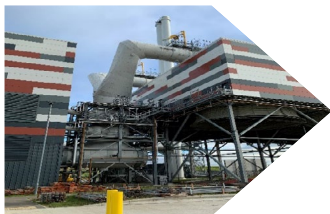
Enfinium Kemsley combined heat and power facility
