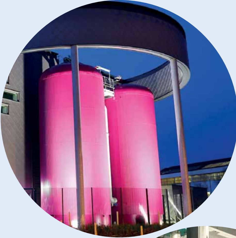
©Gateshead Council and Flexitricity Gateshead Energy Centre
